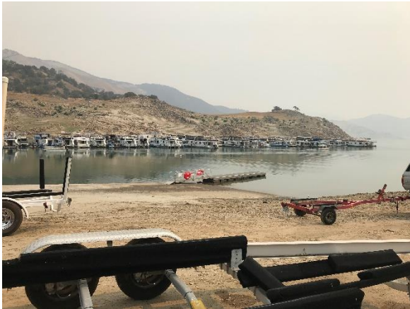
Deer Creek Boarding Float & Boat Ramp
